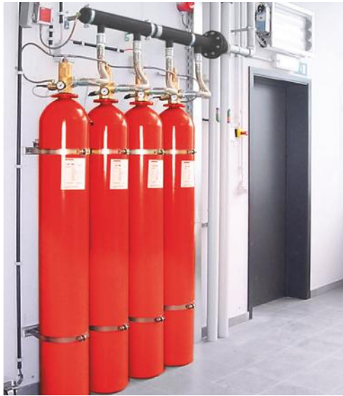
Sinorix 227 provides fast, efficient extinguishing without residues.
